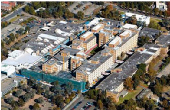
Westmead c2007 – WIN strategy building under construction (Leighton Holdings)
